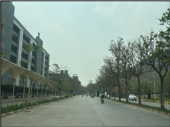
View of the Internal Access Road
