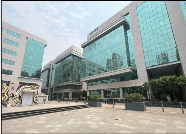
External View of the Subject Property
