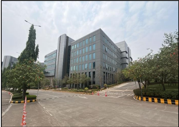
External View of the Subject Property
