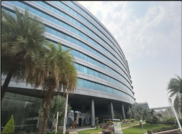
External View of the Subject Property
