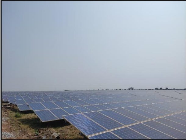
Internal View of the Subject Property
