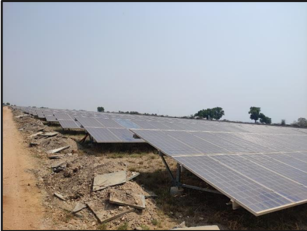
Internal View of the Subject Property
