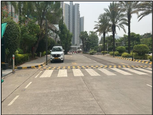
View of the Internal Access Road
