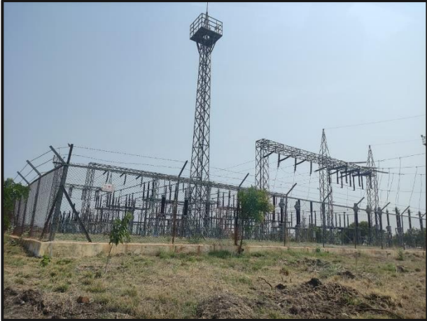
Internal View of the Subject Property
