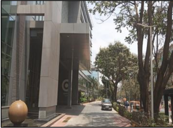
External View of the Subject Property
