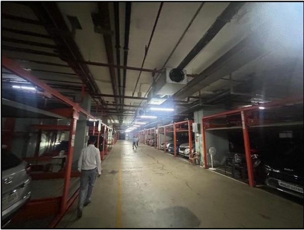
View of the Basement Car Parking
