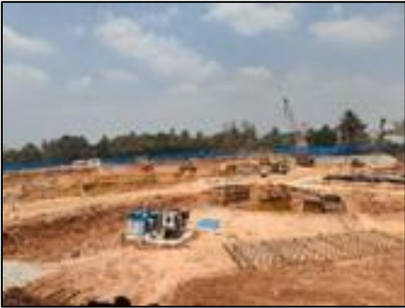
View of the Construction Progress
