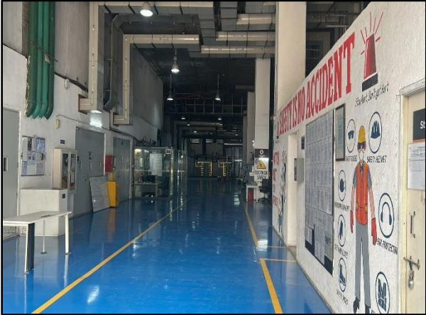
Internal View of the Subject Property
