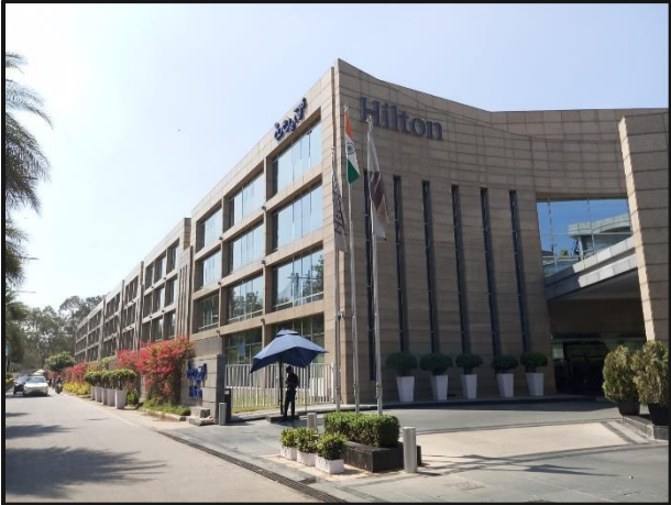
External View of the Subject Property
