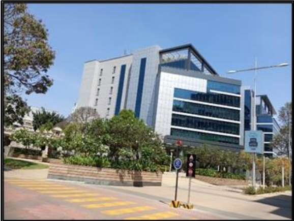
External View of the Subject Property
