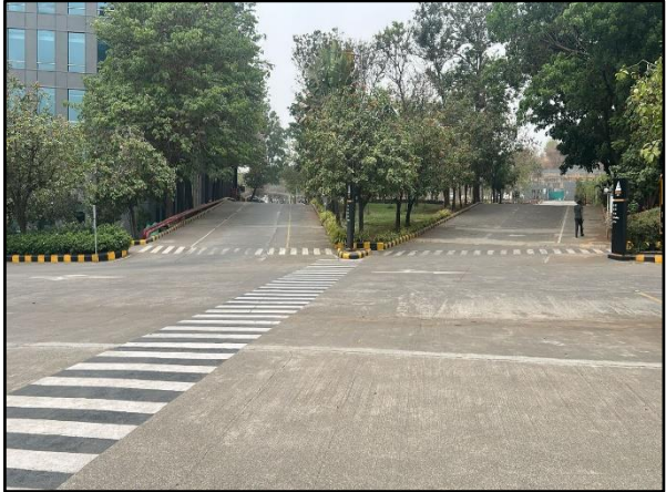
View of the Internal Access Road
