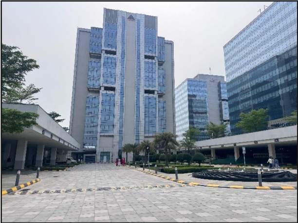
External View of the Subject Property
