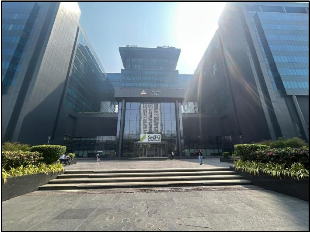
External View of the Subject Property
