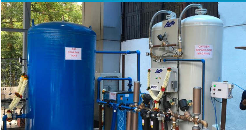
On-site Medical Oxygen Plant (supporting 209 hospital beds )
