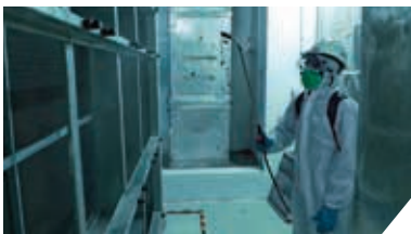
Enhanced AHU Cleaning
