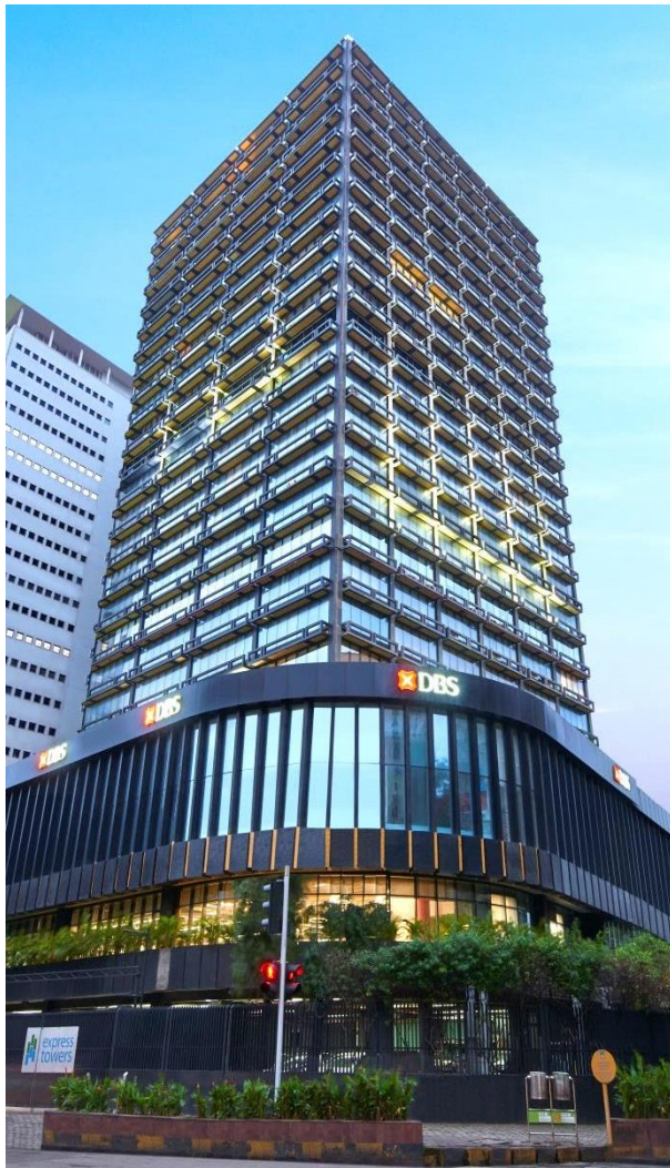
Express Towers Mumbai (0.5 msf)
