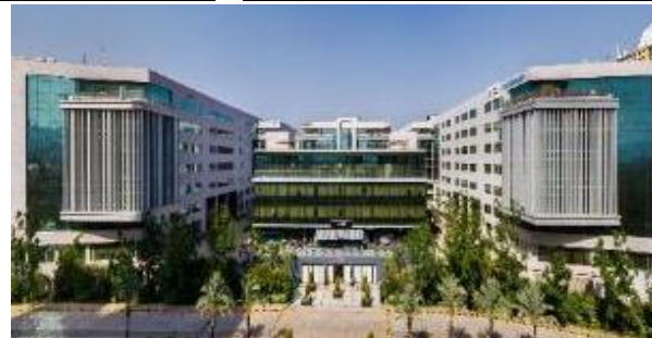
Embassy Qubix Pune (1.5 msf)
