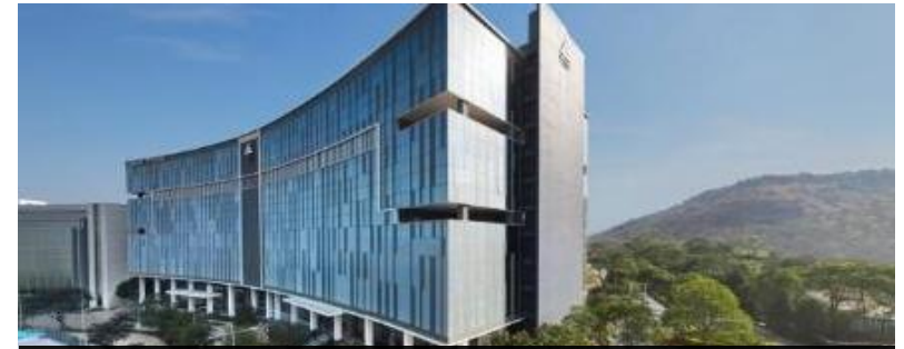
Embassy TechZone Pune (5.5 msf)
