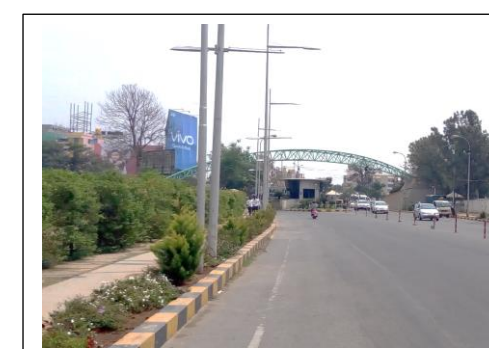
View of the primary access road/entrance
