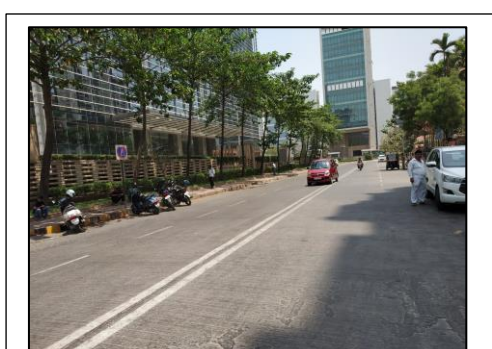
View of Access Road
