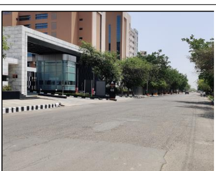
View of the primary access road/entrance
