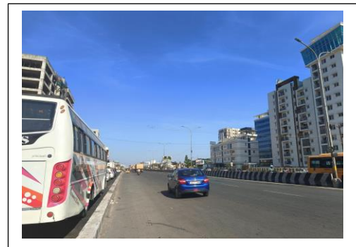
View of the primary access road/entrance
