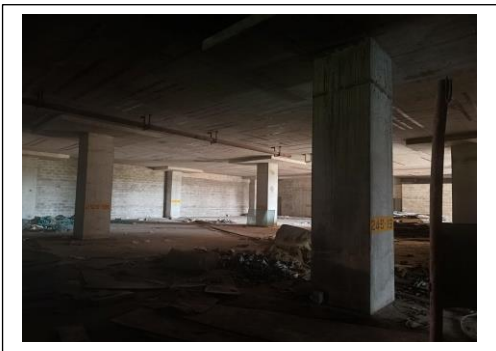
Internal View of the SP
