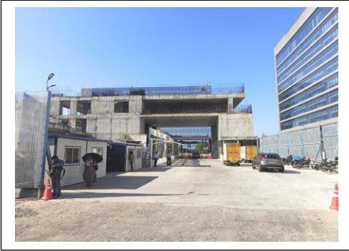
External view of the subject property (SP)
