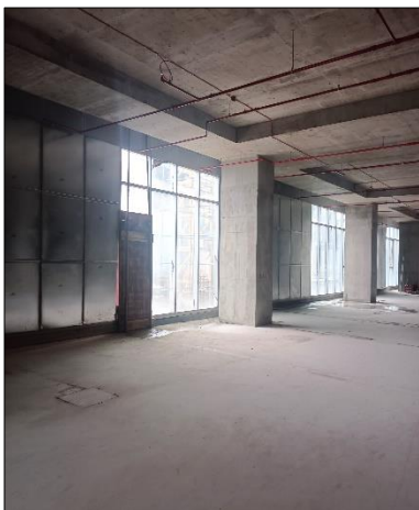
Internal View of the SP
