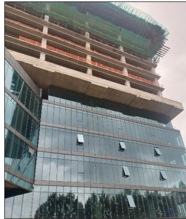
External view of the subject property (SP)
