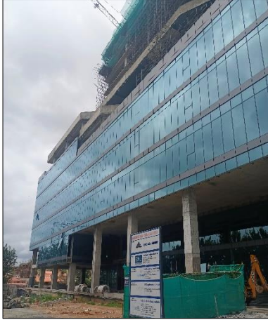
External view of the subject property (SP)
