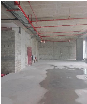
Internal View of the SP
