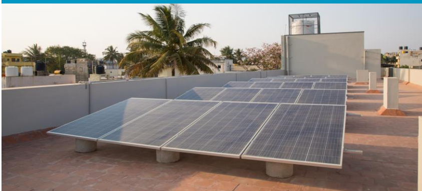
Rooftop solar panel installation to supply green energy (12 schools benefitted)
