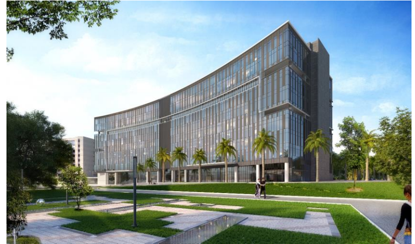
Embassy TechZone – Hudson and Ganges (0.9 msf)
