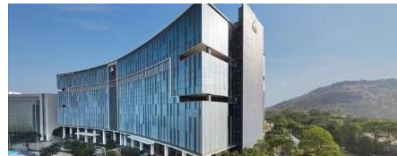
Embassy TechZone Pune (5.5 msf)
